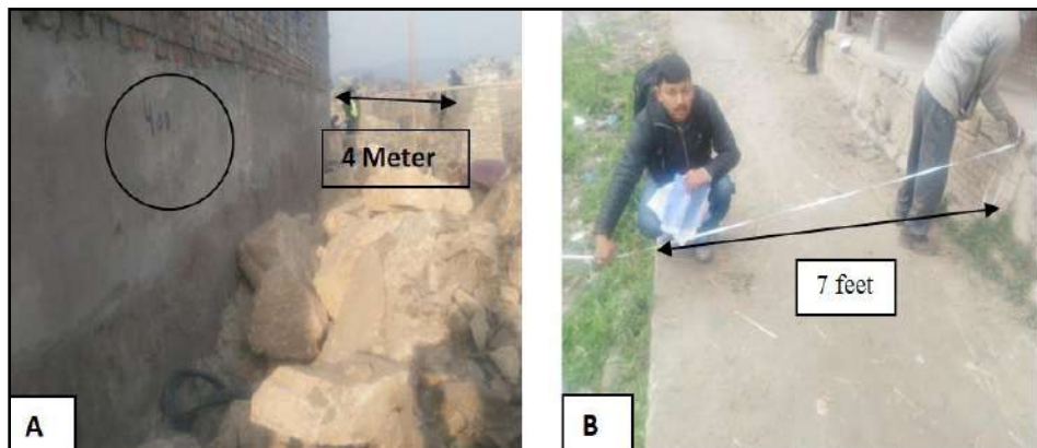
Figure 8: Encroachment by the Garment and Washing Factory (A), Pati build at the Bank of river at Barahisthan (B)
